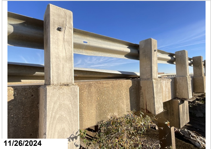
Span 1 has 3 Right posts cracks
